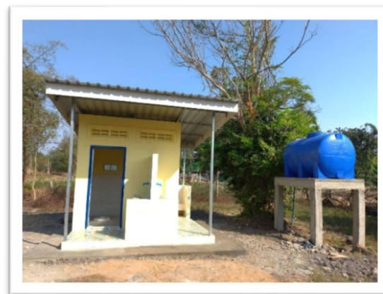
Twin sanitary latrine installed in primary school.
